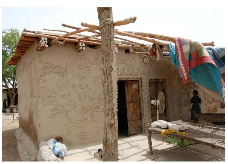
TECHNICALLY SOUND MUD, LIME & BAMBOO Unfired clay walls, extend toe bases, roof projection and strong, accessible KaravanRoof.
