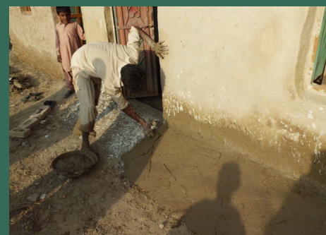
Villagers participating in construction process, making mud toe at the base of the wall.
