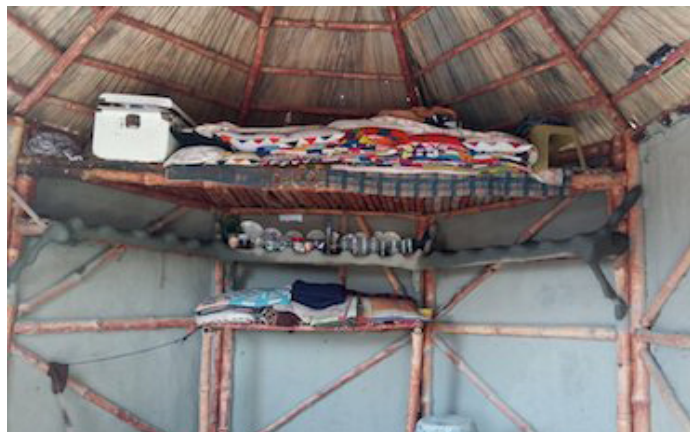
Creation of loft inside the shelter to expand useable space.
