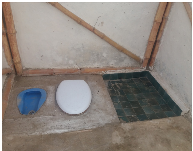
Interior view showing liquid pan, cover with seat, and shower space.
