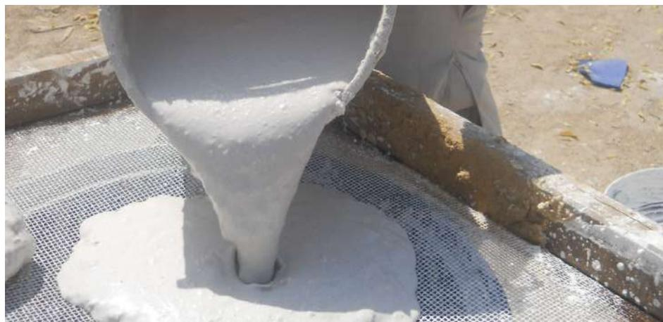
*For a finer finish the lime slurry can be passed through a sieve.*
