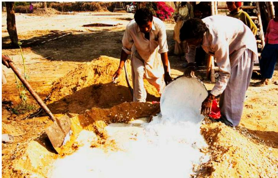
*Mixing slaked lime for laying PLC for foundations.*
