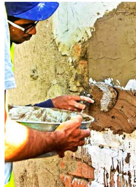
*Different ratios used for plaster produce results of varying strength and colour.*
