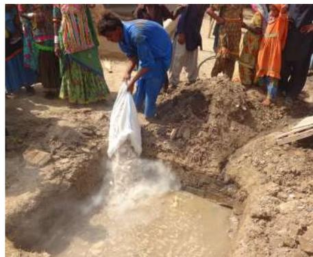
*Ensure that the pit is full of water before adding lime for slaking.*
