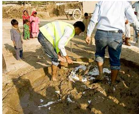
*Mixing straw and dung in mud-lime plaster for wall finishes.*
