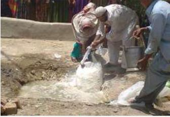
Lime is easily available. It is environmentally friendly as compared to cement. Lime gains strength over time and becomes stronger.
