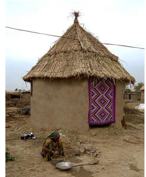
*Lime-mud rendered exterior protects the structure from water damage.*
