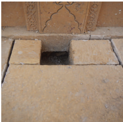
(Far left and left). 'Before' and 'During' images of making up lost stones near drain in the enclosure.
