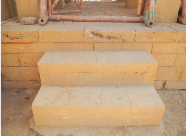
Damaged stone riser at entrance to the canopy.
