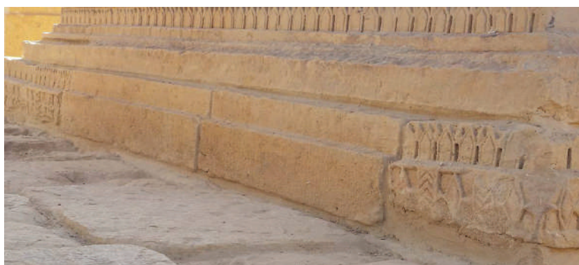
View of sarcophagus after resetting the damaged stones.
