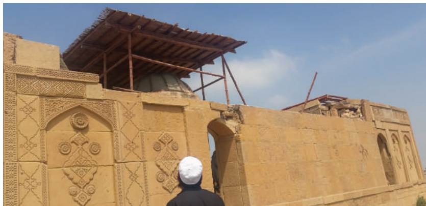
East Perimeter Wall. As part of early 20th c. restoration, rebuilt portion of wall with simple dressed stones between openings can be seen.
