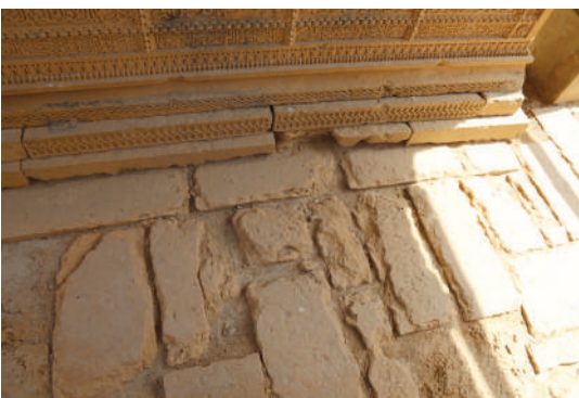
Zenana Chamber. Damaged state of flooring.
