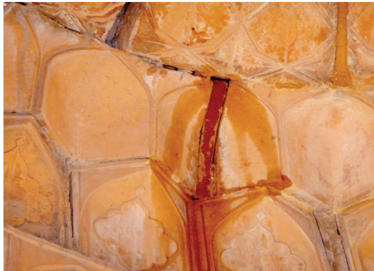
Images recording the process of profiled terracotta infills in large gaps in concentric rings of the extant cupola.
