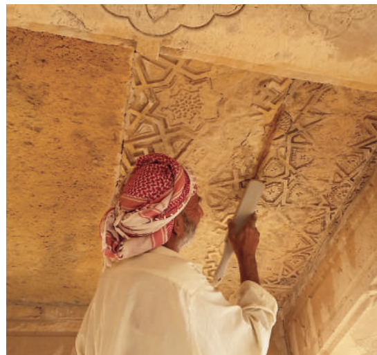
Pointing in gaps of stone slabs of highly eroded roof slabs.
