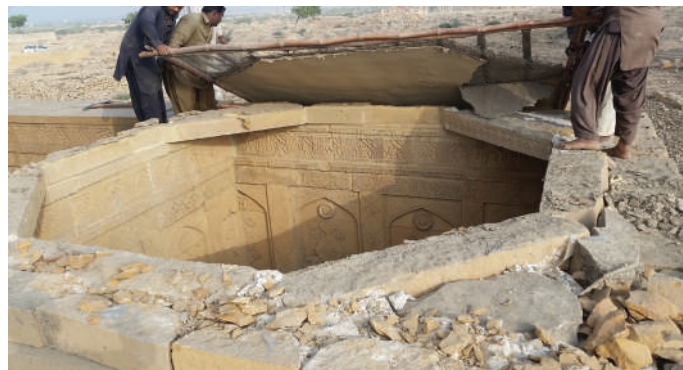
Removing flat bamboo roof to be replaced by bamboo cupola.
