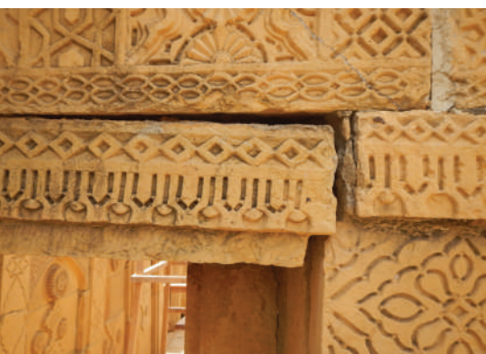
Zenana Chamber. Displaced lintol (above) and view into the chamber (far right).
