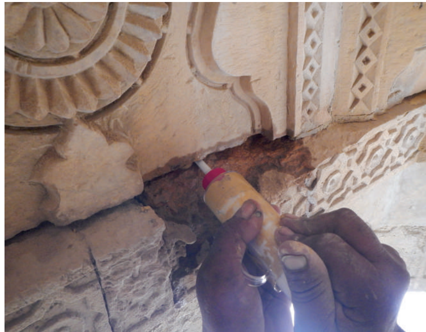
Filling mortar in small joints with an icing gun.
