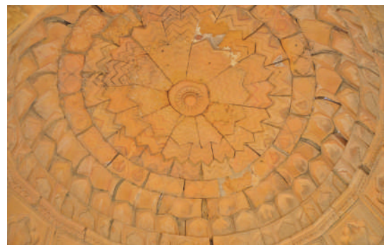
Concentric stone rings in extant cupola.
