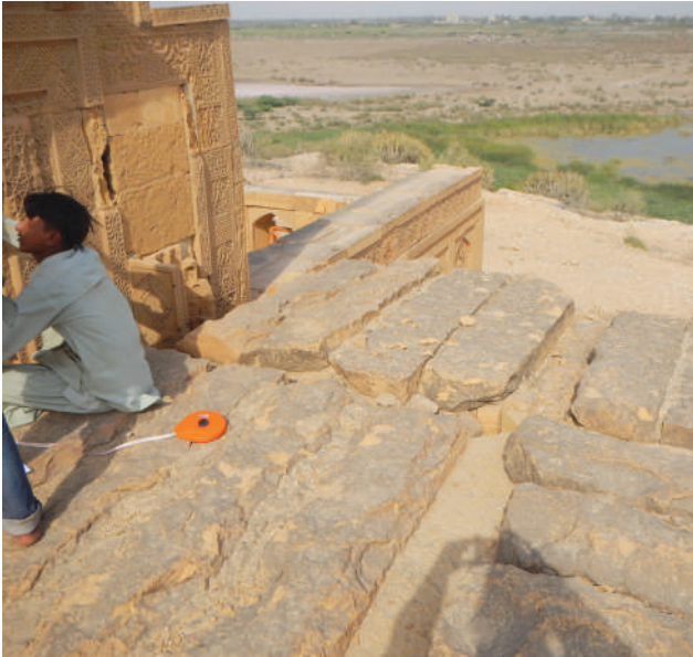
State of joints between damaged roof slabs.
