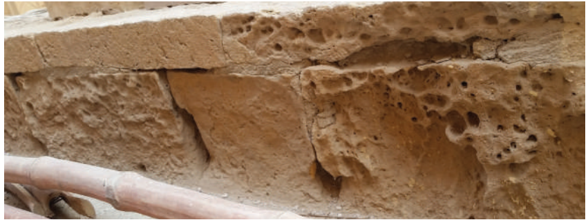
Level of erosion in Graves Platform stones.
