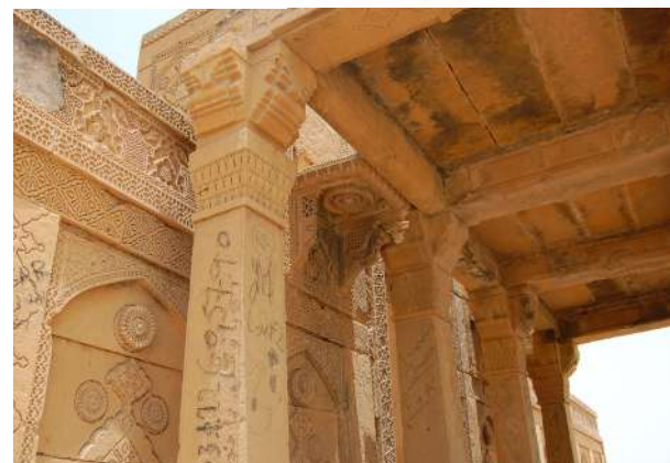
Entrance Canopy. Ravaged roof slabs.
