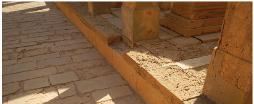
View of stone slabs after injection of mortar.
