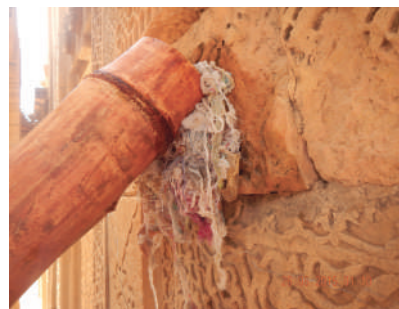
Using poultices to soften dirt.
