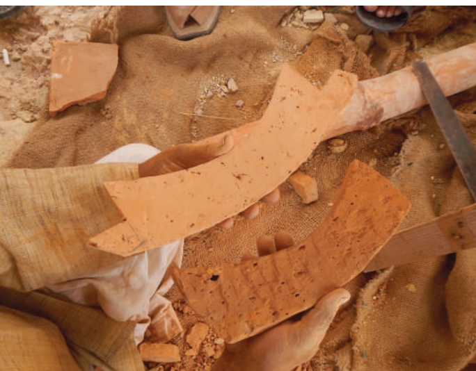
(Above). Stages of profiling terracotta for insertion in dome joints.
