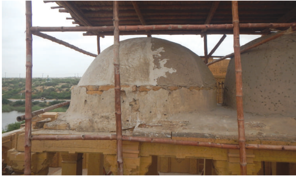
Finishing new dome to match extant central dome.
