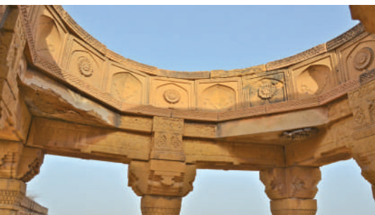
Graves Canopy. Voids show arrangement of phase of transition for cupolas.
