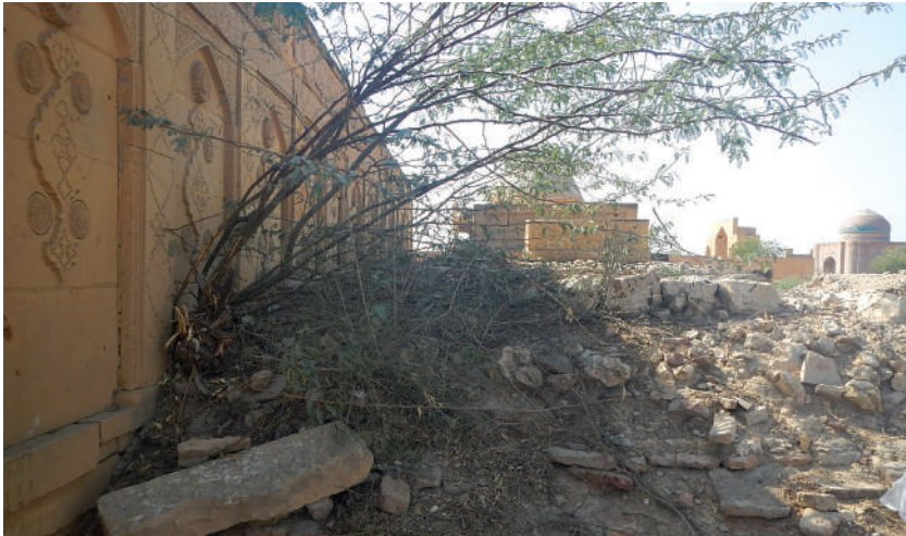
North Perimeter Wall. Grave mounds exerting pressure on the monument wall.
