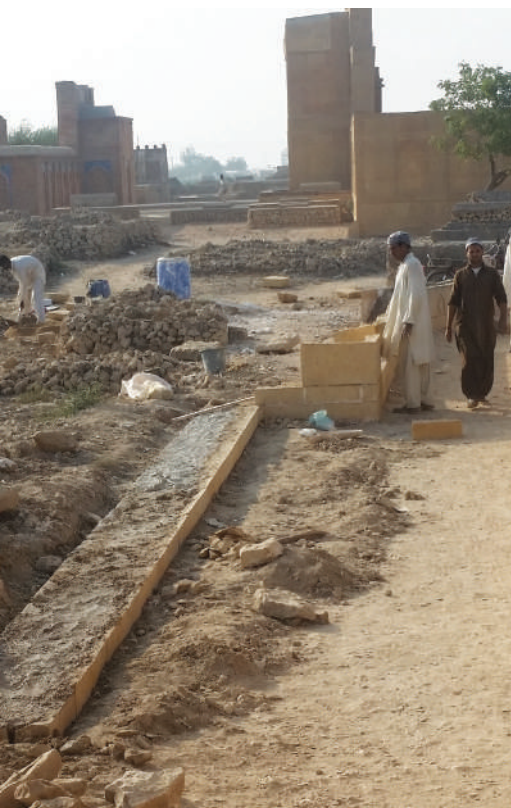
Dwarf wall being restored at east end.
