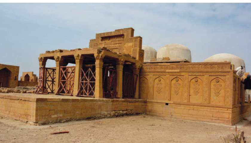
View from southeast. After removing debris and placing unobtrusive plinth protection.
