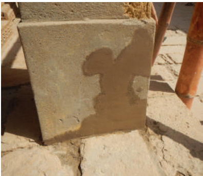
'Before' and 'During' view of sacrificial layer to repair earlier cement intervention.
