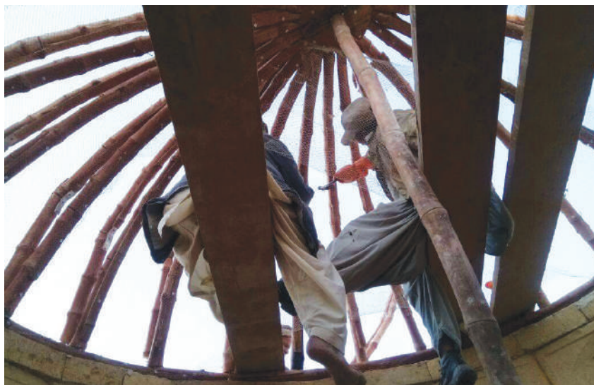
(Above & right) Zenana Chamber. Stages of construction of 2-skeleton bamboo dome.
