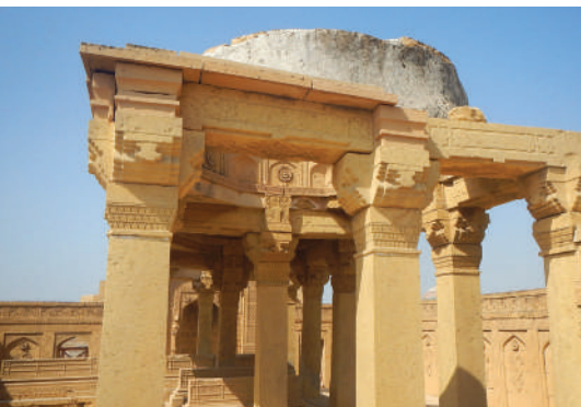
Loss of cupola making structure of Graves Canopy vulnerable.
