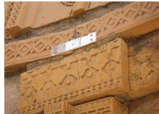
Placement of crack monitors for checking movement.
