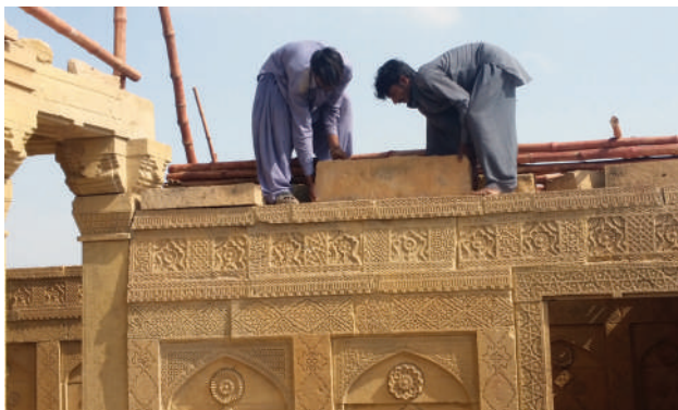
Placing new end pieces to make up loss of stones.
