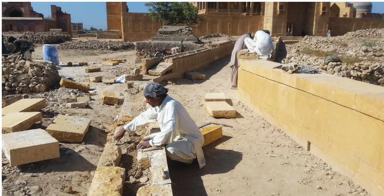
Walkway dwarf wall being restored.
