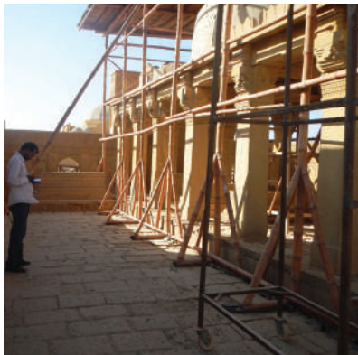
Enclosure. Carefully placed supports for temporary bamboo roof over Graves Canopy.
