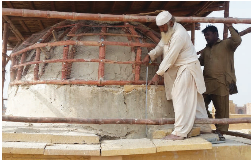
(Right) Ismail Baba constructing double bamboo skeleton with different internal and outer profiles.
