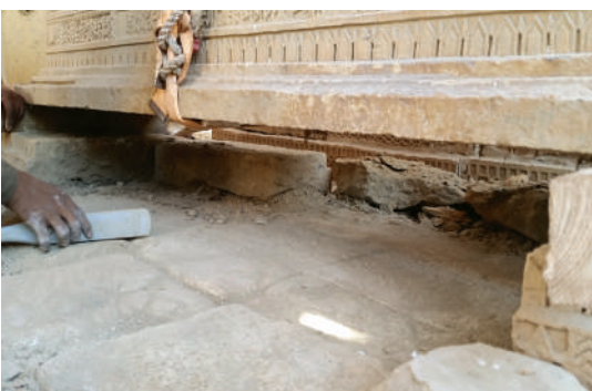
Lifting the sarcophagus to reset eroded stones.
