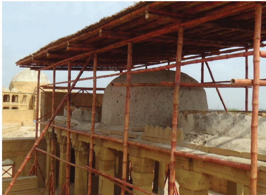
Temporary bamboo roof cover provided to Graves Canopy.
