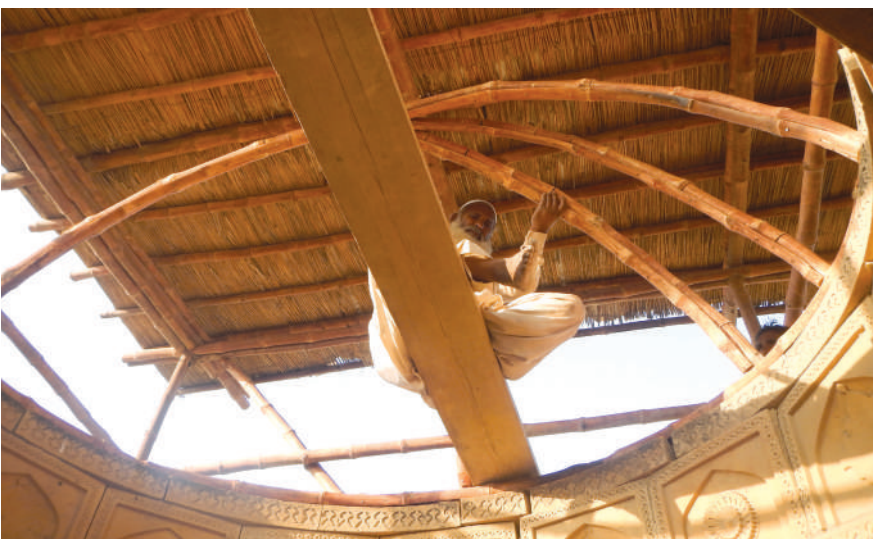
First trial dome on west bay under construction.
