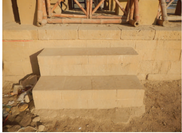
The damaged stone riser at entrance inverted to provide clean edge.
