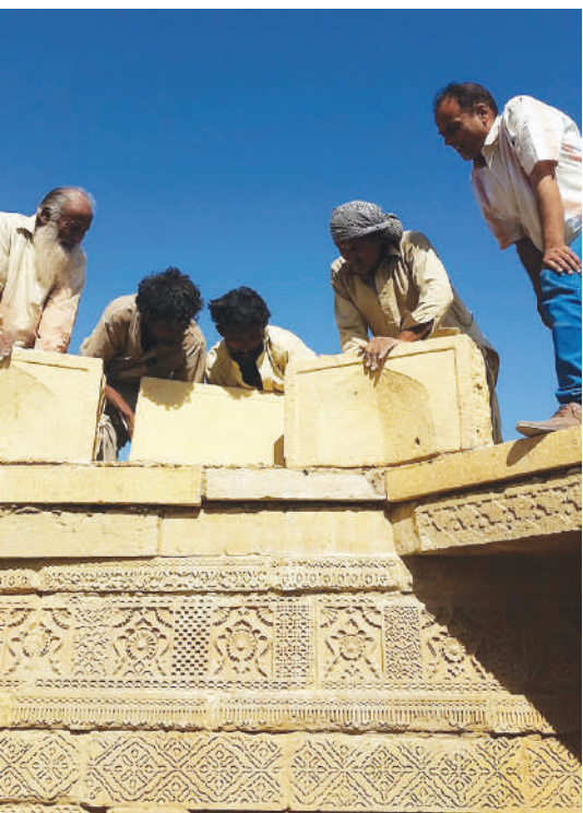
Zenana Chamber. Placement of new stone pieces to form the base for bamboo dome.
