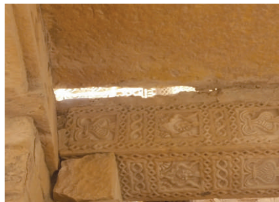
Gaps in roof slabs.
