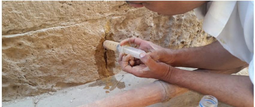
Injecting mortar in voids with sacrificial layer of lime and stone dust.
