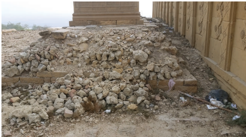
Grave platforms exerting pressure on north Perimeter Wall.
