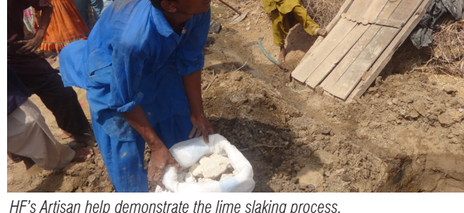
HF's Artisan help demonstrate the lime slaking process.
