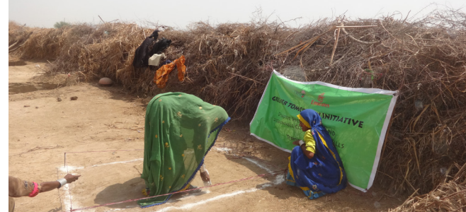
Showing how to measure and mark the structure of Latrine
