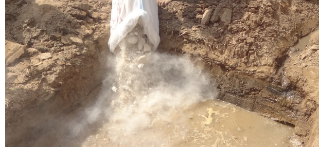
Process of slaking lime being demonstrated
