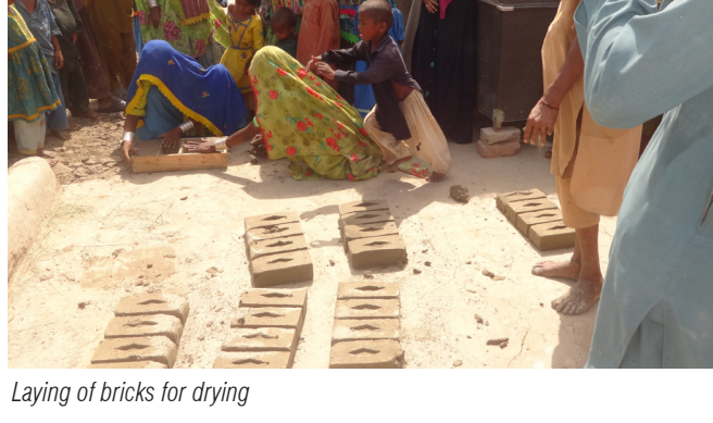
Laying of bricks for drying
