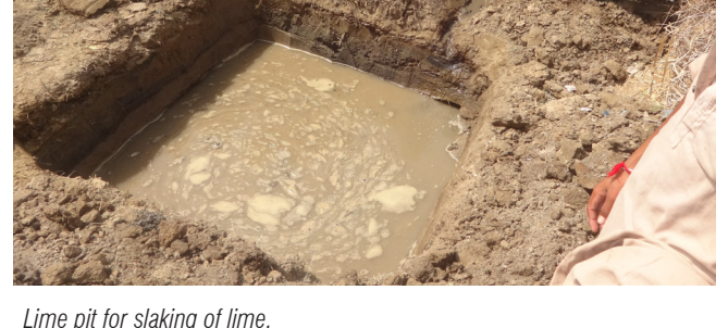
Lime pit for slaking of lime.
