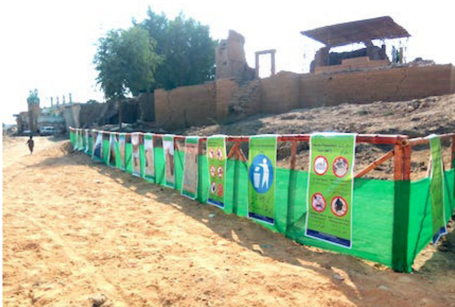
View of Munir Maghfouri tomb site after removal of encroachments. The temporary bamboo roof protects the historic fabric of the mihrab from further damage.
