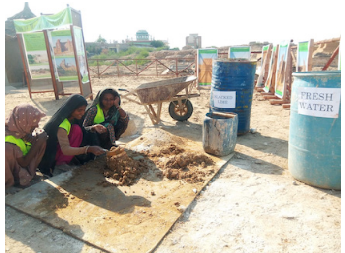
Community women trained for heritage safeguarding mixing lime mortar for use by master masons.
