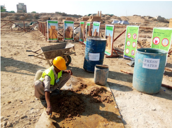
Mason taking freshly prepared mortar for use in underpinning of fragile north wall.
